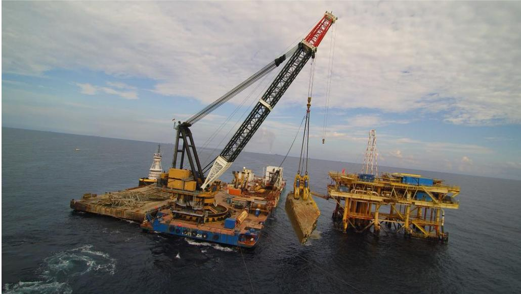
BAY OF CAMPECHE, Mexico (Nov. 15, 2016)- The Conquest MB-1 crane hoists a 600-ton piece of the Troll Solution jack-up wreckage from the Gulf of Mexico. Ardent completed removing the Troll Solution jack-up in November, 2016. This was the largest wreck removal operation in 2016.
